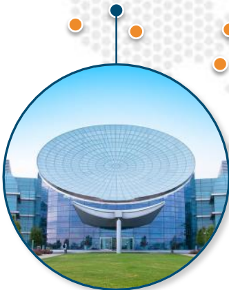
HEADQUARTERS COLORADO USA
